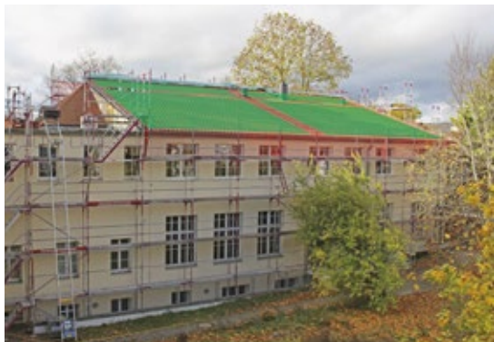
Energy-efficient renovation. The roof surfaces are covered with efficient PVT modules.
